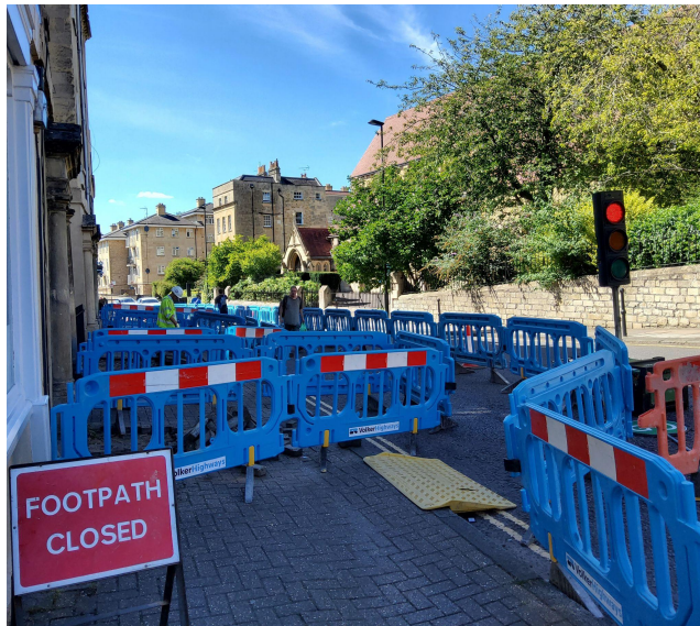
Julian Road pavement repairs underway.
