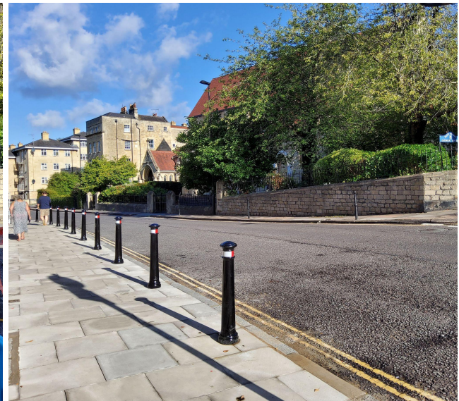
Julian Road pavement repairs completed.
